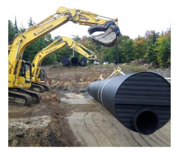
Infra Pipe's Weholite ASTM F894 profile wall structural polyethylene system provides a 100-year design life and is resistant to H2S, pH, corrosion, and abrasion. Weholite has been used throughout the world and North America since 1981.
